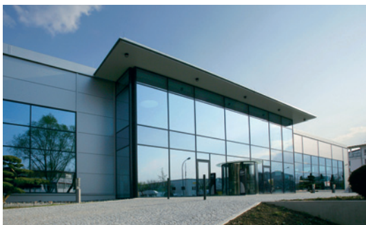
Figure 4: Zahoransky AG, Systems Technology plant in Freiburg, Germany.
