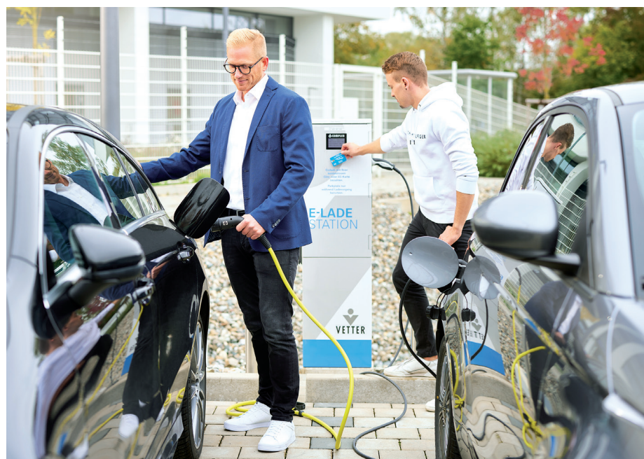
Figure 2: Allow employees to charge their EVs at onsite charging stations.
