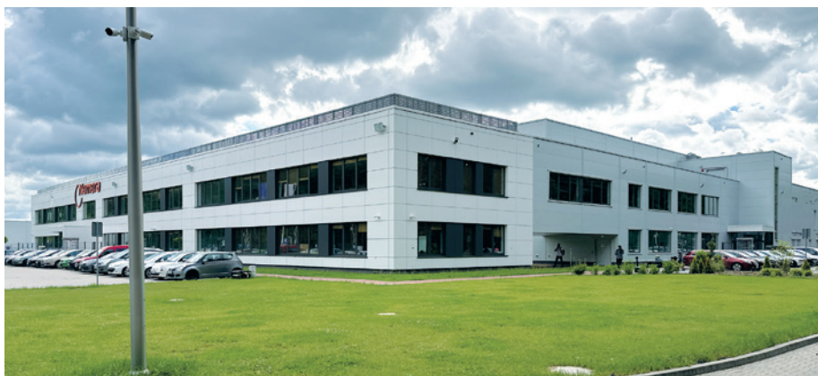
Figure 4: State-of-the-art facility dedicated to pen injector manufacturing in Szczecin, Poland.
